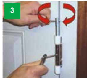
When in position secure the socket screw. **Take care not to overtighten.** Replace the covers.
