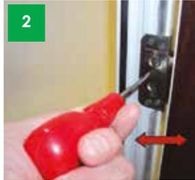
Lever the slide plate (B) with a screwdriver in the adjustment slot.
