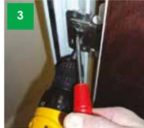
Secure the screws in the side plate.
