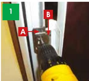
1 Remove the 2 screws that clamp side plate (B) to frame plate (A) to all three hinges
