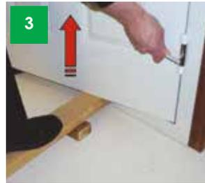
Lift and support the door to the required height whilst securing the socket screws. **Take care not to overtighten.** Replace the covers.
